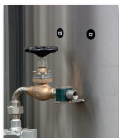
Gas use point ready for connection
